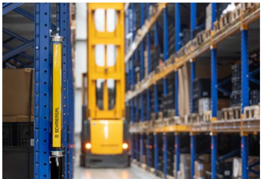
Fig. 1: In intralogistics systems, alternative wiring concepts for safety switchgear offer particular benefits.
