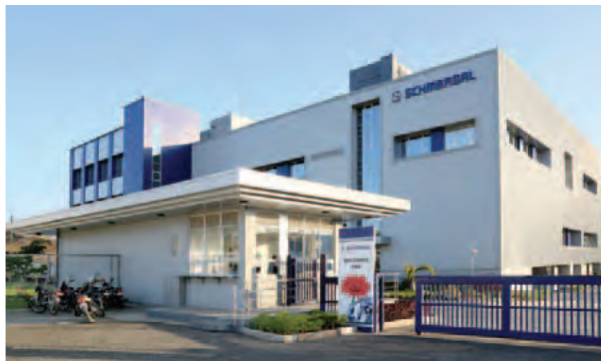
The Schmersal factory in Ranjangaon started production in July 2013.
