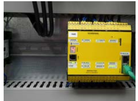
Fig. 2: The PROTECT PSC1 safety controller is always used when the customer requires a “safety separated” safety concept.
