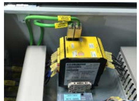
The decentralised safety solution with the PSC1 safety controller from Schmersal reduces the wiring required.
