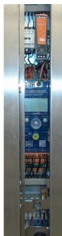
Figure 34: The control cabinet are supplied as installed in control cabinets for wall mounting, as floor standing cabinets or in door frames.
