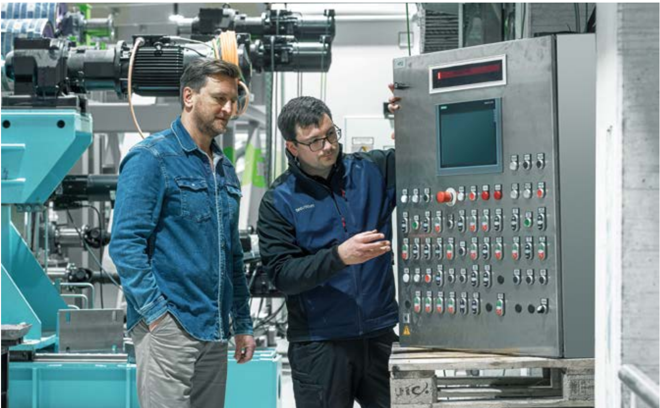
The IIoT solution 'Energy Management Solution' creates the conditions for optimising energy consumption in production.
